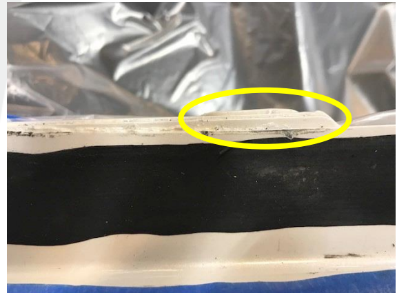
Figure 4 – Uneven sheet metal overlap, overhead view (windshield removed)
