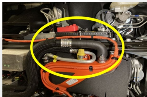
Figure 4- Foam Installed (Europe)
