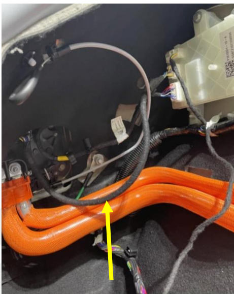
✓ Figure 10 – Wiring harness is correctly routed in front of busbars
