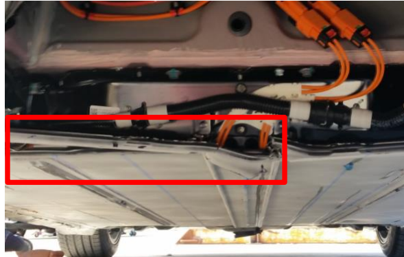
Figure 9 – Torn front skid plate
