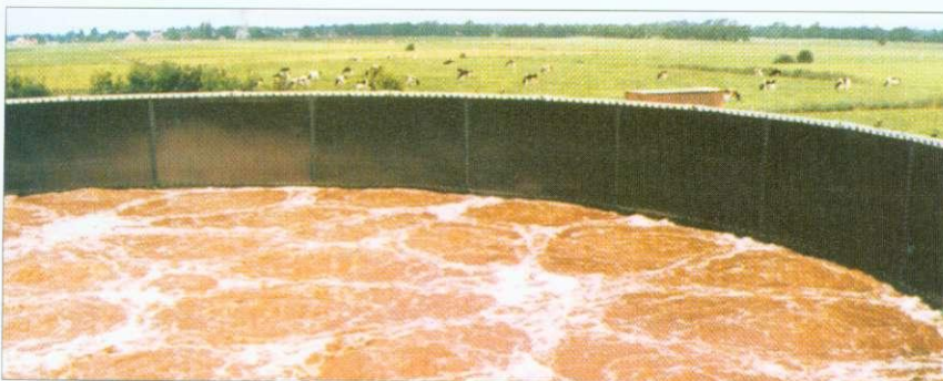
An oxidation tank that treats polluted waste water
