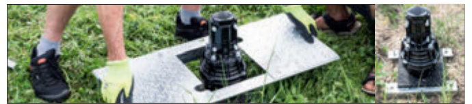
Fig. 14: Base plate with YAESU G-1000 SDX
