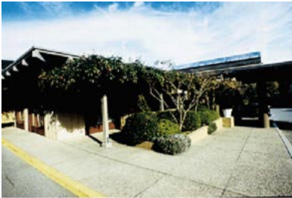
Fig. 11 Trellis with vines provides shade for south side of building.
