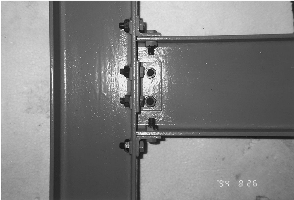
Figure 10. Beam-column connection.
