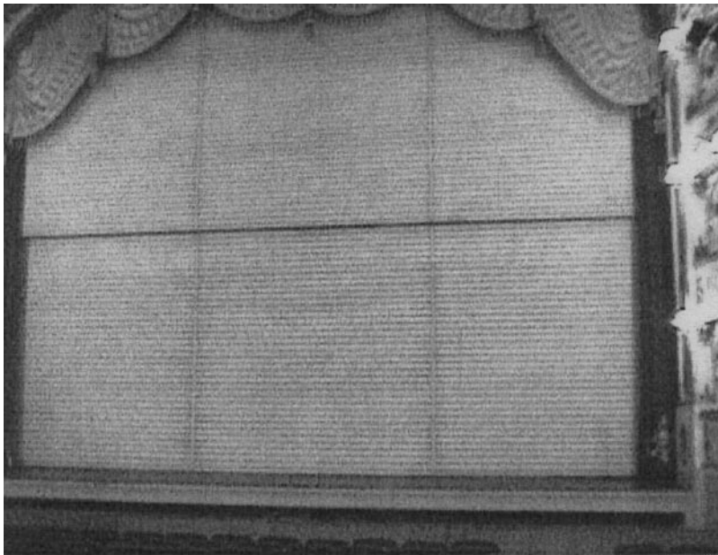
Figure 11. View of the fire-curtain from the hall.
