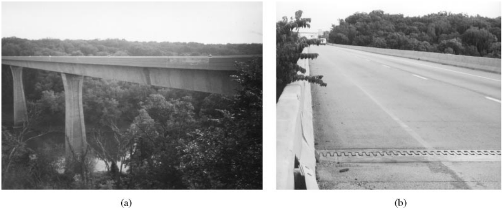
Figure 8. Views of (a) the Kiswaukee bridge and (b) top deck.
