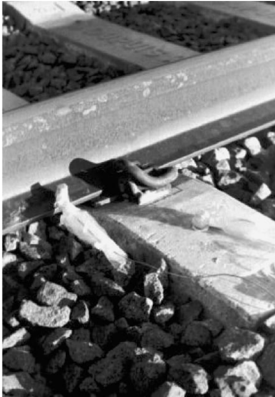
Figure 6. Accelerometers glued to the rail and sleeper of track 2.
