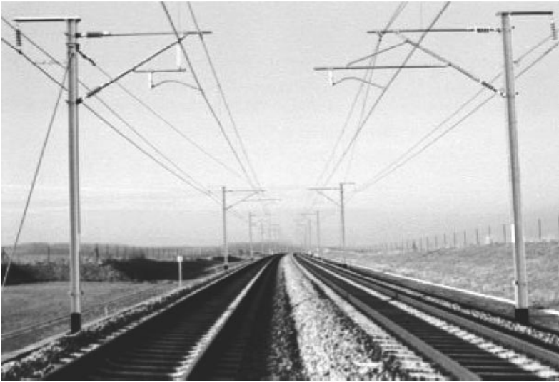
Figure 2. The HST track between Brussels and Paris.
