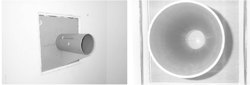
Fig. 13. Photograph of duct taken from receiver room looking into the duct.
