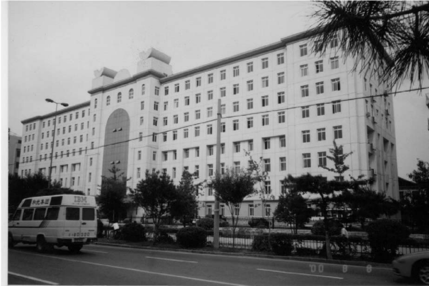
Fig. 9. Practical building photograph of the story-increased structure after construction.
