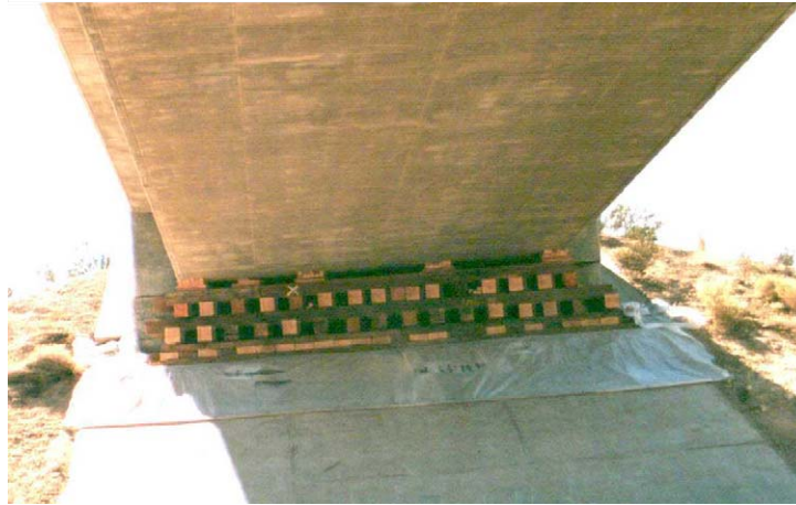
Fig. 4. A view of temporary shoring installed under the bridge superstructure.
