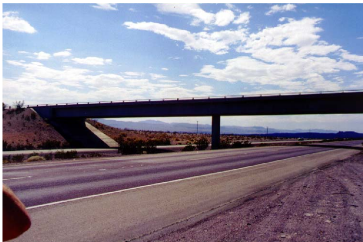
Fig. 1. View of the Lavic Road Bridge.
