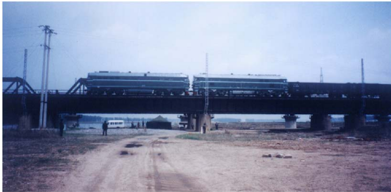
Fig. 1. Experiment site at Daqinghe Bridge.
