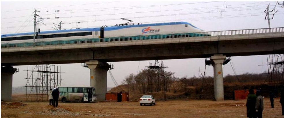
Fig. 1. Field test of Gouhe River Bridge under China-Star high-speed train.
