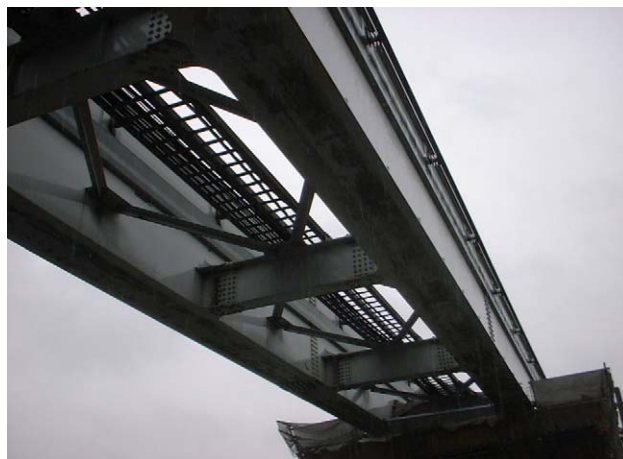
Fig. 1. View of the monorail steel bridge.
