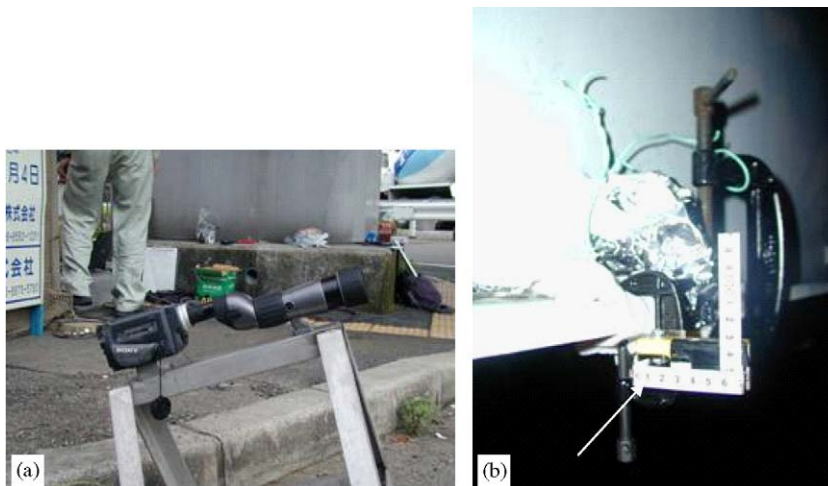
Fig. 6. Installation for field-test of monorail bridge: (a) video camera equipped with telescope and (b) measuring target for displacement.
