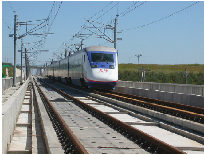
Fig. 9. Pioneer Train running on the Gouhe Bridge.
