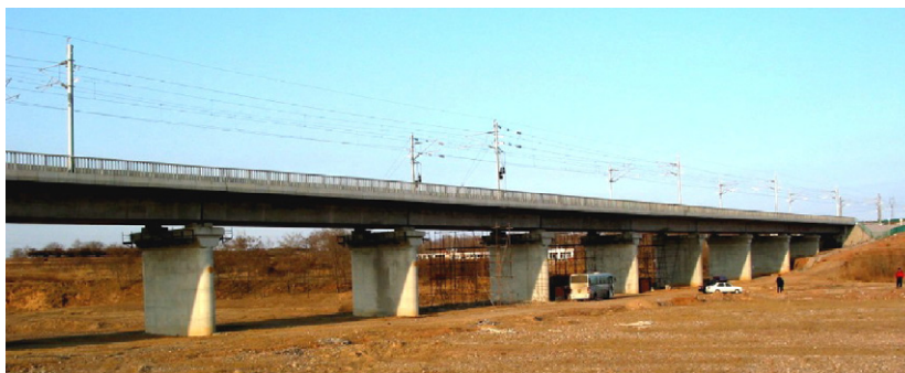
Fig. 5. View of the Gouhe River Bridge.
