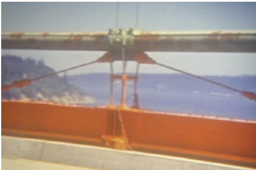
Fig. 2. Diagonal ties and midspan cable band (from Washington State Archives, with permission).
