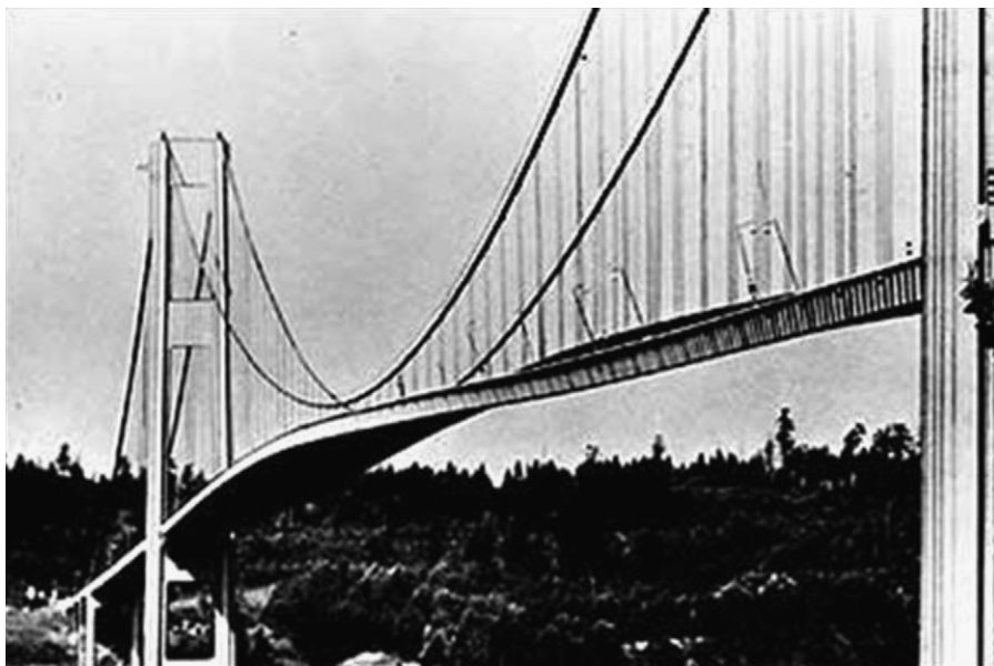
Fig. 1. Torsional motion on November 7, 1940 (from Ref. [9], with permission from Washington State Department of Transportation; GHPHSM, Bashford 2784).
