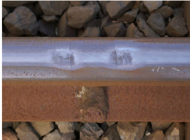
Fig. 19. Squats in the hardness minima in the heat-affected zone at the surface of an aluminothermic rail weld.
