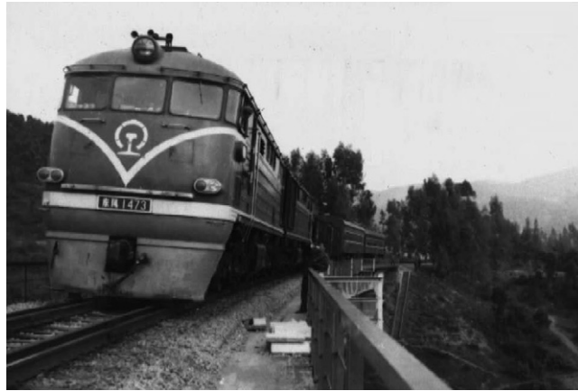
Fig. 8. Test train on the Xihe Bridge during experiment.
