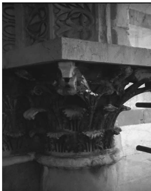
Fig. 2. Capital of the Baptistery of Piazza dei Miracoli in Pisa where black crusts are clearly evident.
