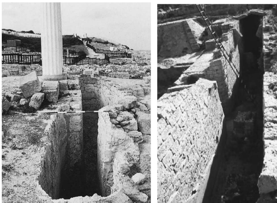
Fig. 1. Typical aspect of the cisterns of Tharros. In particular, the cisterns 3 and 5 are shown on the left and right sides, respectively. The mortar samples were mainly taken from the upper parts of the cistern walls at about 100 cm from the bottom wall level. Because the sampled Phoenician–Punic cisterns of Tharros are generally characterised by a height variable from 1.80 to 2.5 m, the sampled areas were located at about half distance from the bottom level and the roof of the cistern. Furthermore, the cisterns are characterised by an elongated shape with a width ranging from 1 and 1.5 m and a length that varies from 3 to about 5 m.
