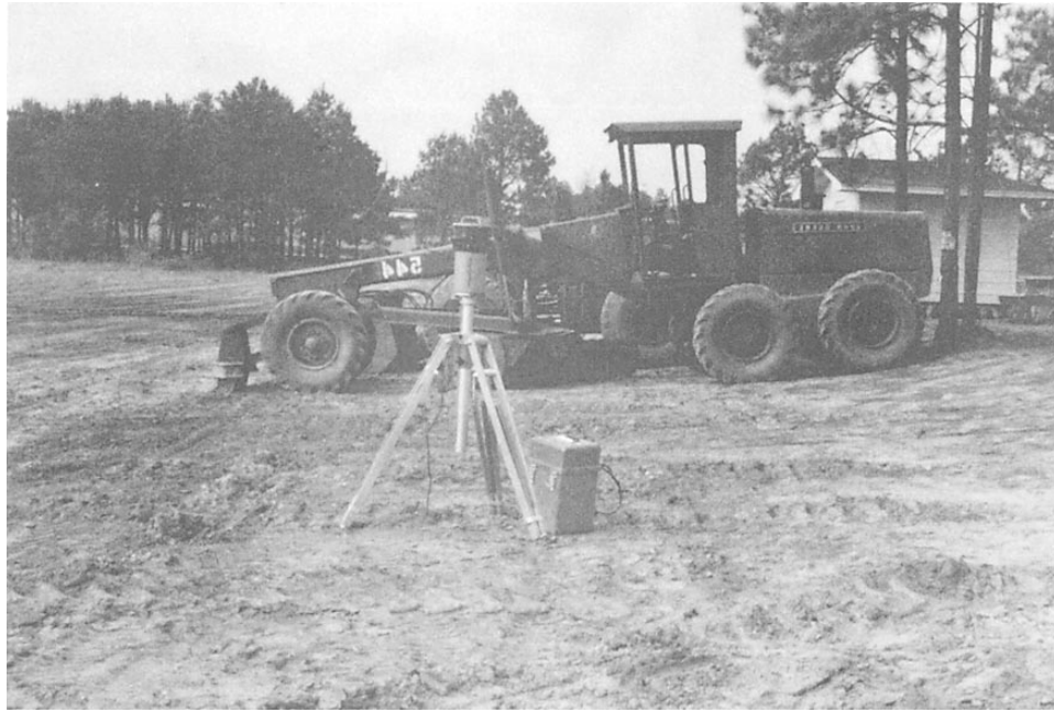
Figure 12-8.—Grading machine controlled by laser level and laser detector.
