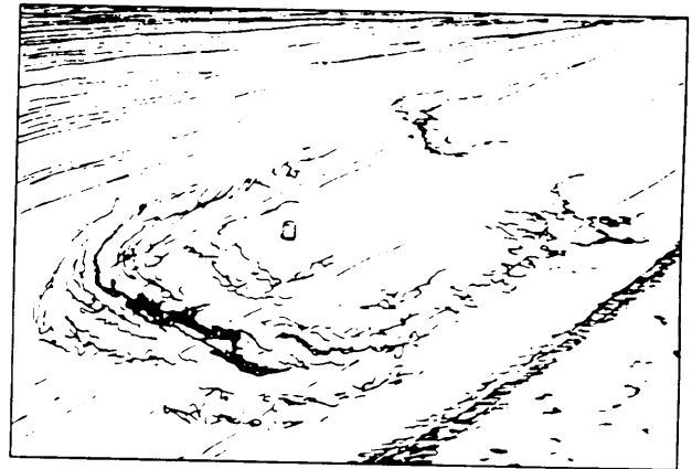
Figure 16-15.-Slippage cracks.
