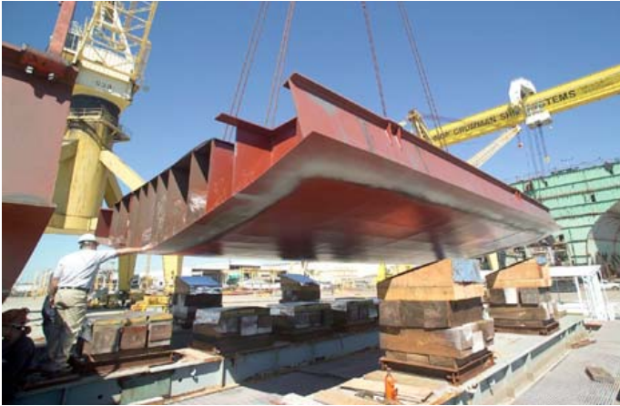
Newly assembled keel for the first Deepwater National Security Cutter (WMSL-750) was displayed at the Keel Laying event on March 29, 2005.
